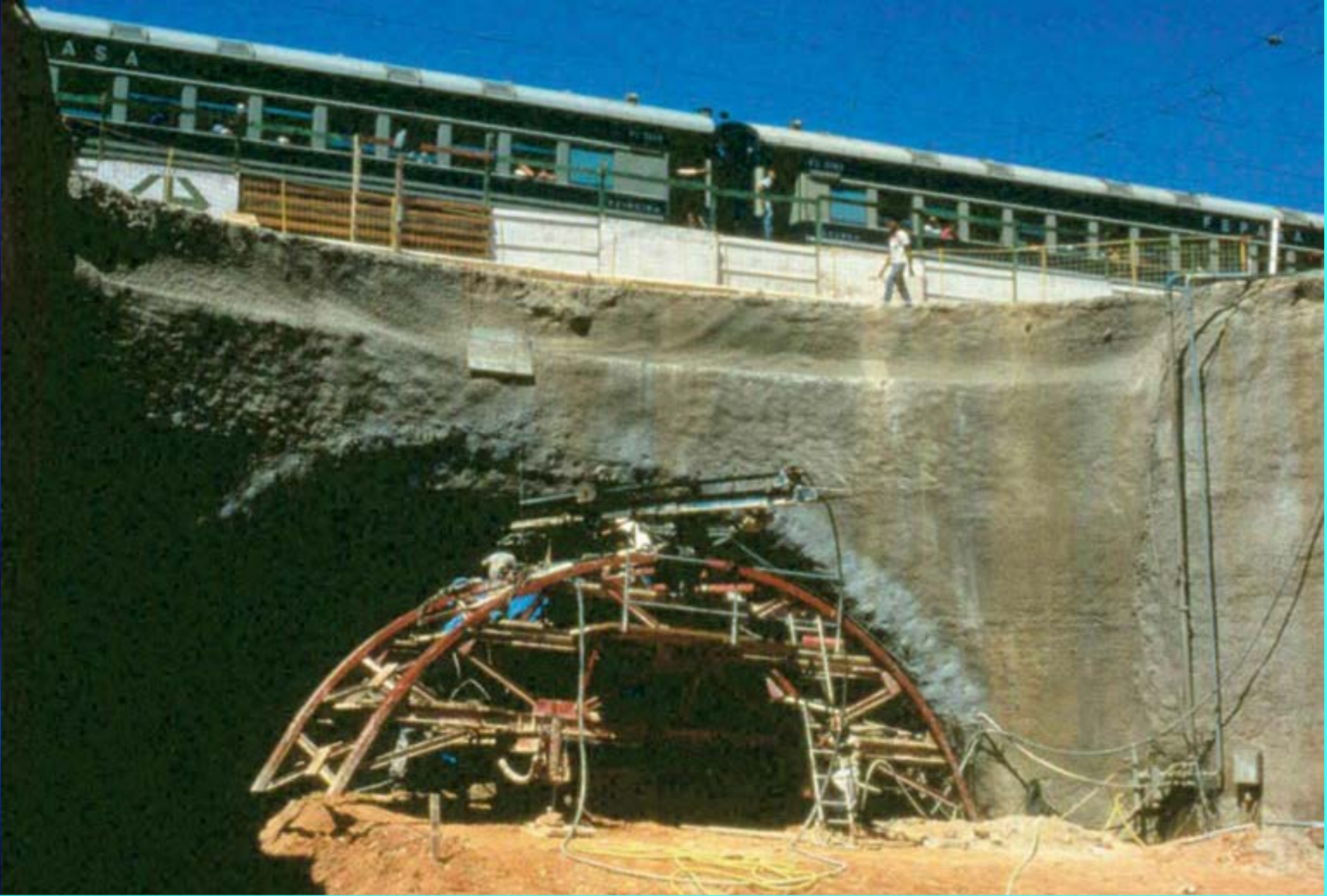
View of the portal constructed using a shell of ground improved by means of jet-grouting and face reinforced with jet grouting elements. In Campinas (Brazil) [Lunardi Proyect]
