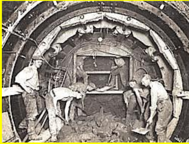
Hydraulic Shield (Fig, 1.3) Steinway Tunnel, 1907 (now Queensboro Tunnel)
